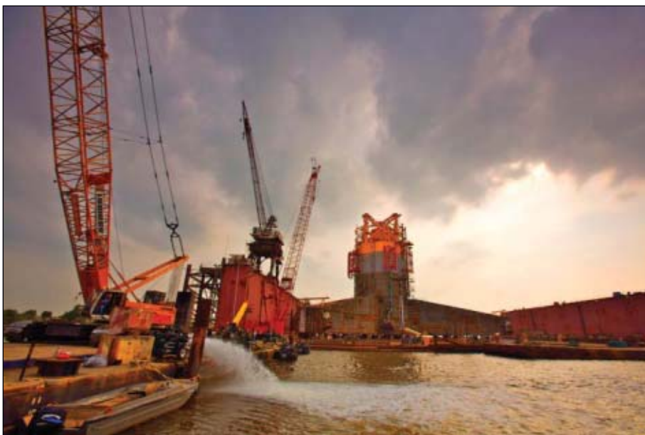
The Neptune SeaStar monocolumn tension-leg platform hull has been under construction in the Signal International dry dock yard, Port Arthur, Tex. (Fig. 1; photo from BHP Billiton Petroleum Americas Inc.).
